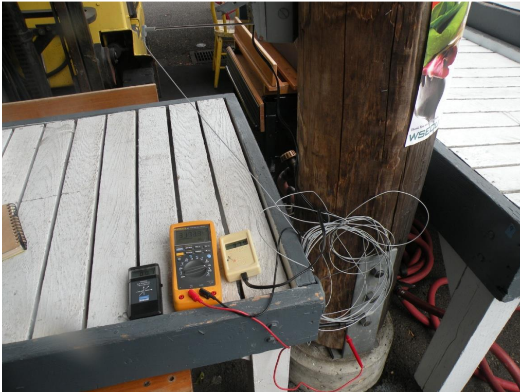
Figure 2 Amperage between outlet ground and metal support
